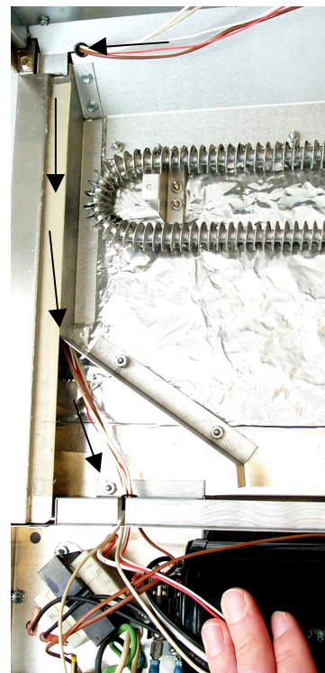
Figure 4: The hi-limit is shown mounted on its standoffs.
